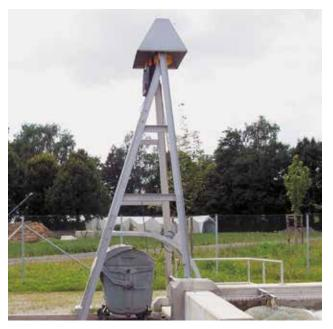
On the HUBER Basket Screen CageLift, the electromechanical lifting mechanism is mounted above the channel or pump shaft, so that the screenings can be discharged directly into a container.
