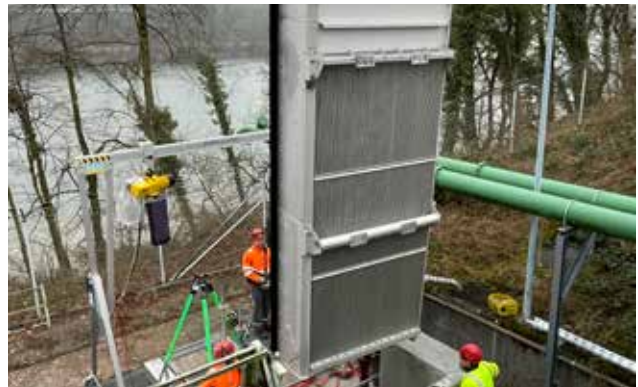
Installation of a RakeMax® during plant modernisation.
