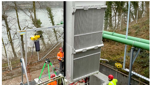
Installation of a RakeMax® V during plant modernisation.
