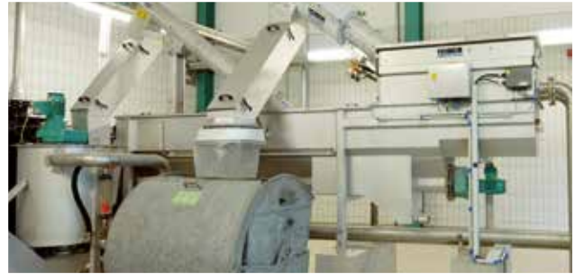
Well-proven mechanical pre-treatment components combined within the HUBER Sludge Acceptance Plant ROTAMAT® Ro3.3.
