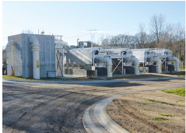
4 HUBER Disc Filter RoDisc® with 18 discs in stainless steel container.
