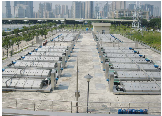
28 HUBER Disc Filter RoDisc® units with 24 discs each treating about 8.5 m 3 wastewater per second.
