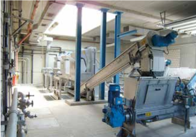
3 HUBER Fine Screen STEP SCREEN® SSV units: L=4300, W= 1176, 3 mm slot width. Optimally adjustable to suit specific constructional conditions (big discharge heights, deep channels) due to the steep installation angle of 70° to 80°.
