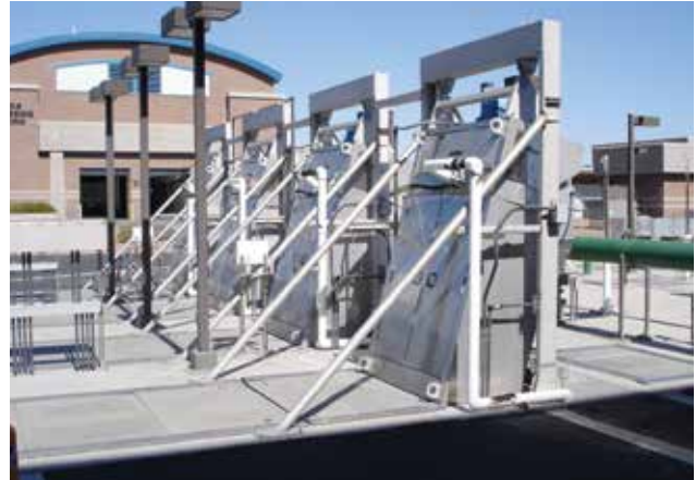
4 HUBER Fine Screen STEP SCREEN® SSV units: L= 5300, W=1376, 6 mm slot width, installation angle 75°. Maximum operational stability due to the special bottom step design for increased operational reliability without impairment by grit, gravel, stones.
