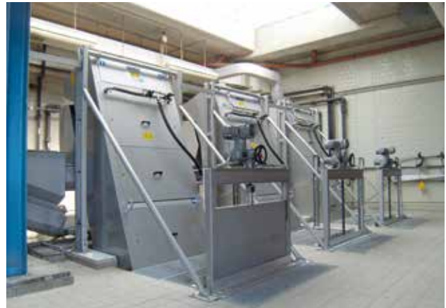
HUBER Fine Screen STEP SCREEN® SSV: 4300 mm long, 3 mm slot width, acid treated in a pickling bath for optimal corrosion protection.
