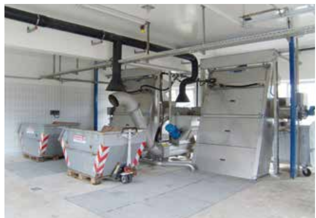
Two HUBER Fine Screen STEP SCREEN® SSV units, length 4300 mm, width 1676, 6 mm slot width, combined with HUBER Wash Press WAP® type SL for intensive screenings washing. Totally enclosed, odour-free design.
