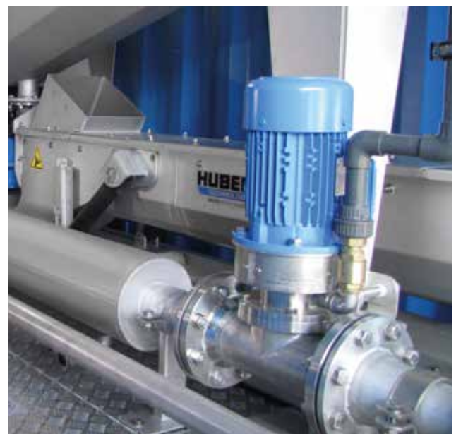
IPM 100 installed upstream of sludge dewatering system.
