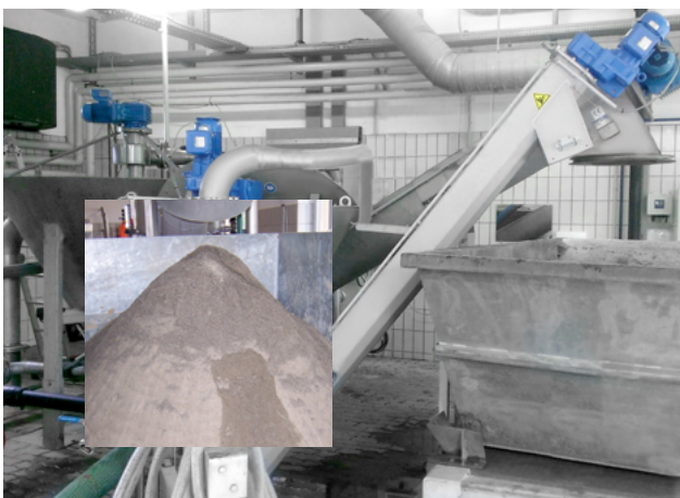
Grit washer installation on a municipal sewage treatment plant.
