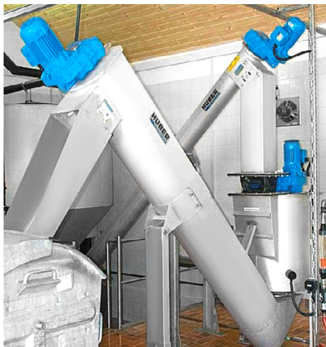
The HUBER Grit Washer RoSF4 T washes the classified grit from a HUBER Circular Grit Trap HRSF.
