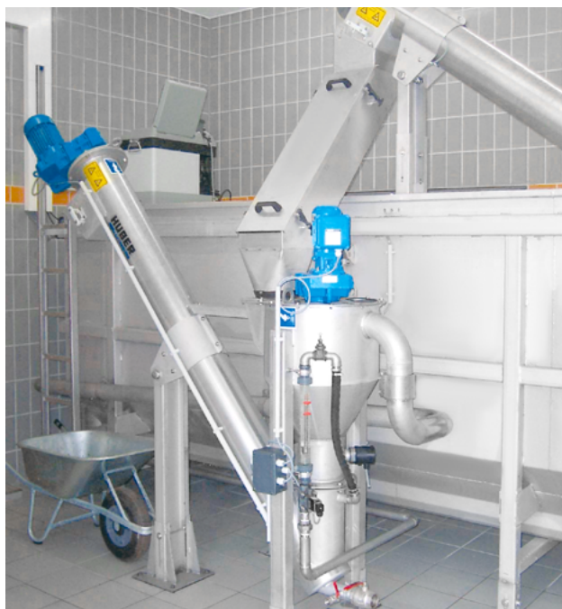
A small HUBER Grit Washer RoSF4 TC washing the classified grit from a HUBER Complete Plant ROTAMAT® Ro5.
