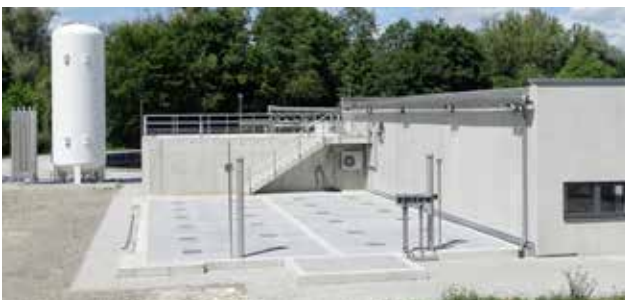
Concrete basin variant of the HUBER Active Carbon Filter CONTIFLOW® GAK.
