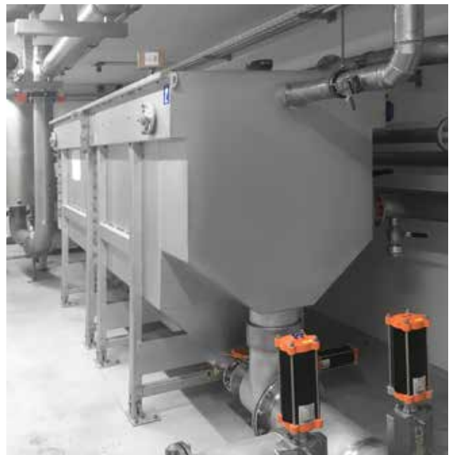
HUBER Heat Exchanger RoWin for heat recovery and wastewater cooling – energy optimisation and compliance with temperature limits.
