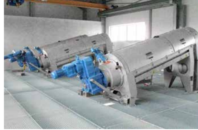
HUBER Screw Press units for sludge treatment – best dewatering performance and highest volume reduction for lower disposal costs.
