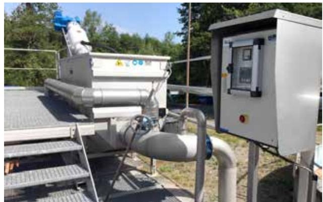
*Process wastewater screening for textile fibre separation.*
