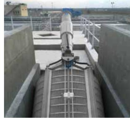
*HUBER Perforated Plate Screen ROTAMAT® STAR for protecting downstream membrane filtration systems.*
