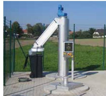
*HUBER Pumping Stations Screen ROTAMAT® RoK4 with heating for outdoor installation.*
