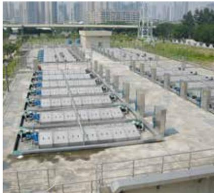
24 installed HUBER Disc Filter RoDisc® units.
