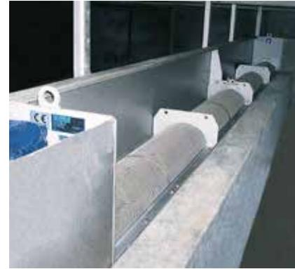
*HUBER Storm Screen ROTAMAT® RoK2 installed on four side of overflow weir.*
