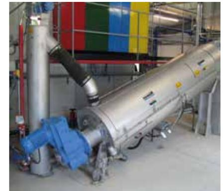
HUBER Screw Press S-PRESS: specific power consumption < 0.01 kWh/kg<sub>DR</sub>.
