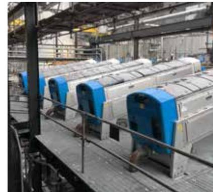
*Sludge dewatering with HUBER Screw Press Q-PRESS® 800.2.*
