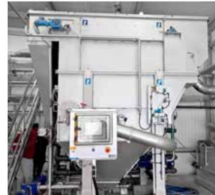
*HUBER Dissolved Air Flotation Plant HDF for internal water recycling.*
