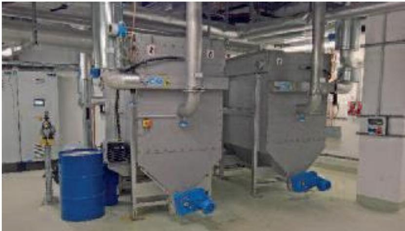
**Fig. 31: Wastewater heat utilisation – the Museum “Haus der Bayerische Geschichte” (pictured above) in Regensburg uses the HUBER ThermWin system with the HUBER Heat Exchangers RoWin (pictured below) to heat and cool the building. This replaces fossil fuels with renewable wastewater energy.**
