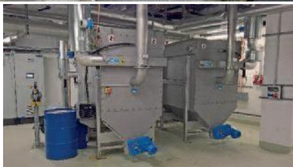
Fig. 36: Wastewater heat utilisation – the Museum ‘House of Bavarian History’ in Regensburg (pictured above © Picture documentation, City of Regensburg) uses the HUBER ThermWin system with the HUBER Heat Exchanger RoWin (pictured below) to heat and cool the building. This replaces fossil fuels with renewable wastewater energy.
