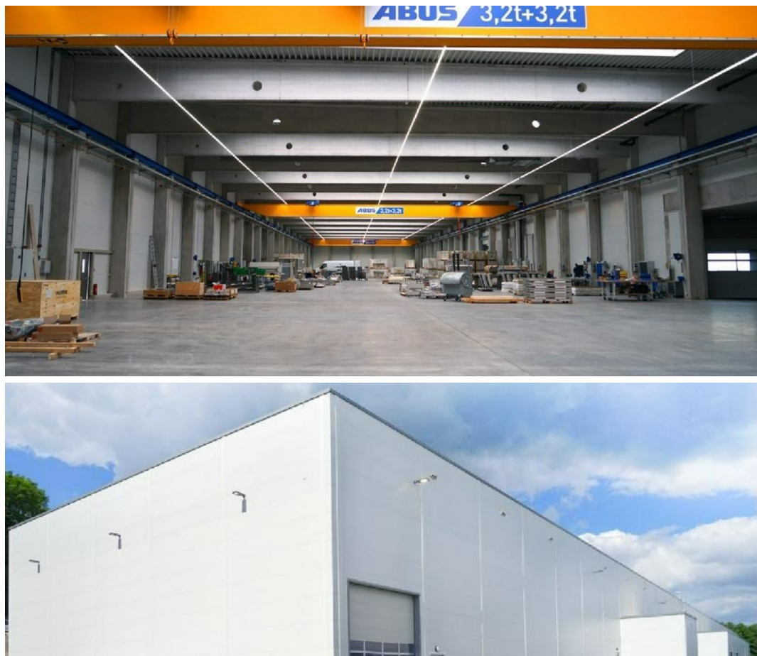
Fig. 20: The new 5,500 m 2 assembly and logistics hall P4 was completed and commissioned in 2024.
