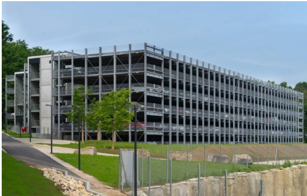
Fig. 47: The car park was built in 2024 and has been used by all HUBER SE employees since April 2025.
