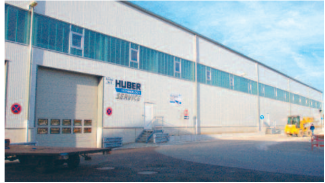
HUBER repair service factory
