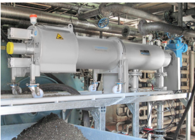
HUBER Sludge Cleaner STRAINPRESS® integrated into the pipeline (Great Britain).
