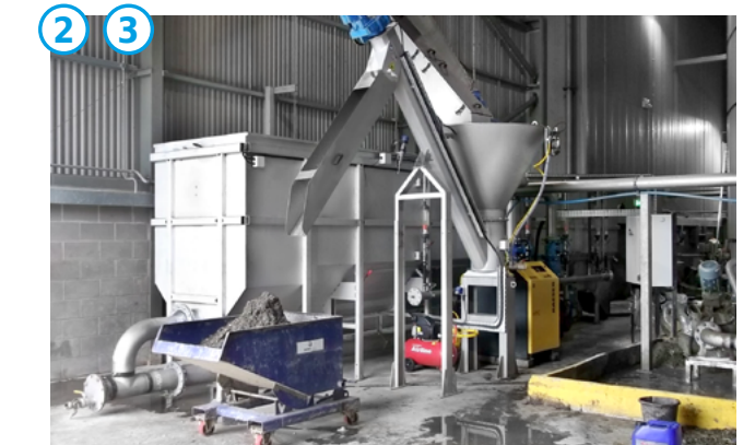
HUBER Longitudinal Grit Trap ROTAMAT® Ro6 Bio and HUBER Grit Washing Plant RoSF G4E Bio.
