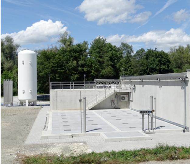
24 HUBER Active Carbon Filter CONTIFLOW® GAK with upstream ozonisation.
