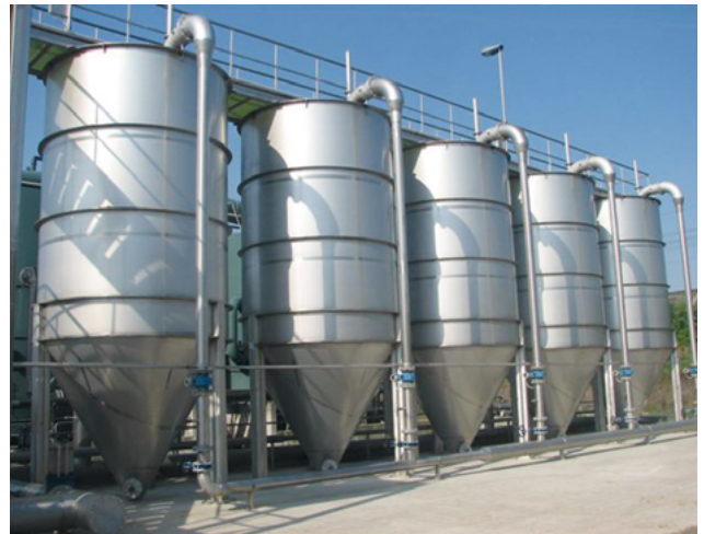
HUBER Sandfilter CONTIFLOW® 72, Montebello, Italy.
