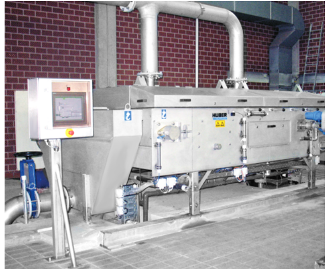
HUBER Belt Thickener DrainBelt for up to 100 m 3 /h thin sludge.
