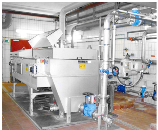
HUBER Belt Thickener DrainBelt for 60 m 3 thin sludge per hour.
