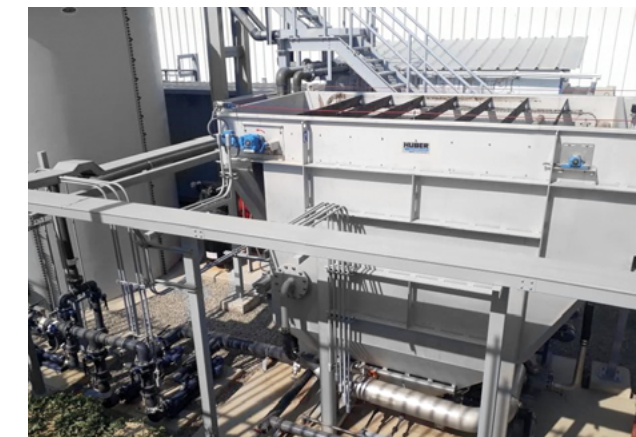
HUBER Dissolved Air Flotation for physical-chemical pre-treatment – optimum reduction of COD, fats and solids, more than 500 installations worldwide.
