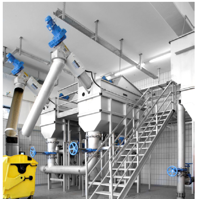
HUBER Rotary Drum Fine Screen ROTAMAT® Ro2 with high-pressure cleaning – best cleaning results and adapted machine technology.
