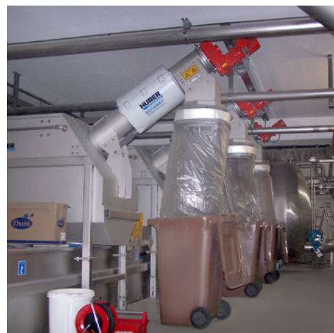
HUBER screens and fine screens as well as grit and heavy material separators for the best possible and project-specific mechanical treatment of wash water and production wastewater from – efficient, durable, tried and tested.
