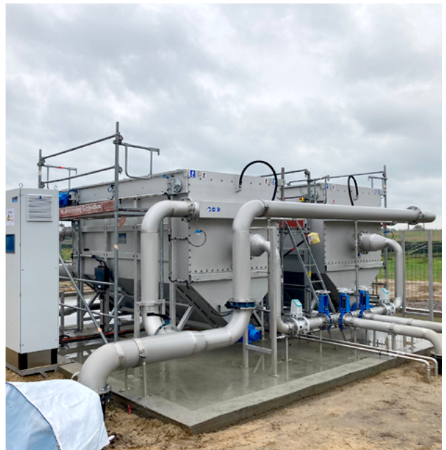
HUBER Wastewater Heat Exchanger – energy recuperation and wastewater cooling.
