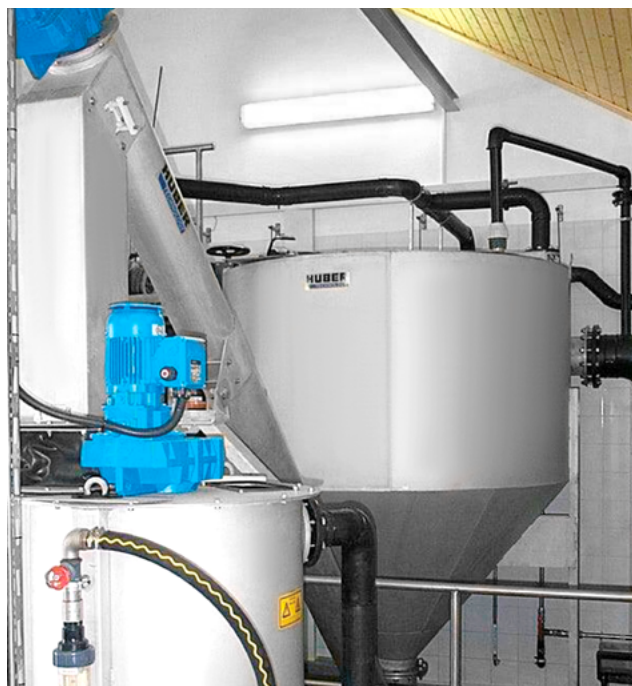
HUBER Circular Grit Trap HRSF with integrated classifying screw and subsequent HUBER Grit Washer RoSF4 T.
