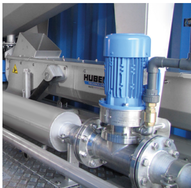
IPM 100 installed upstream of sludge dewatering system.
