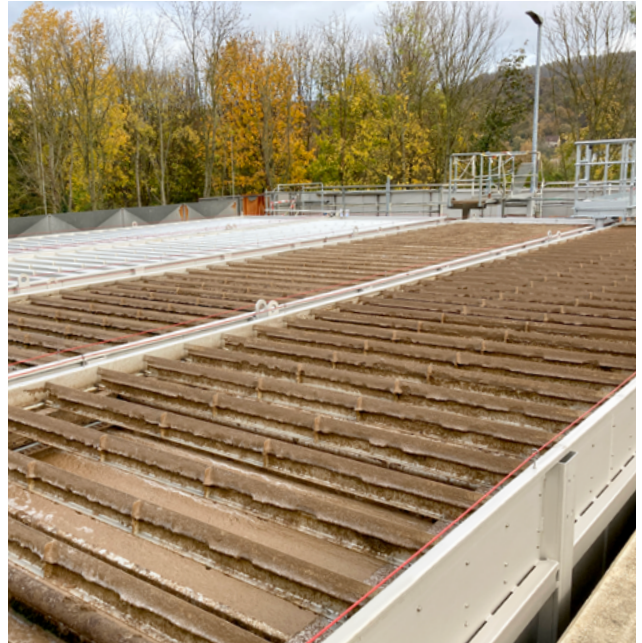
HUBER Dissolved Air Flotations Plants with chemical stage for secondary treatment – the solution to relieve overloaded biological treatment plants.
