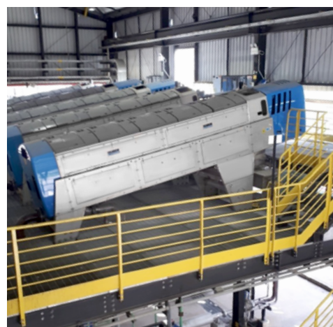
HUBER Screw Press units for sludge treatment – best dewatering performance and highest volume reduction for lower disposal costs.
