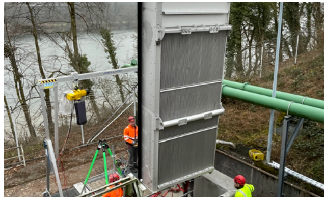
Installation of a RakeMax® during plant modernisation.
