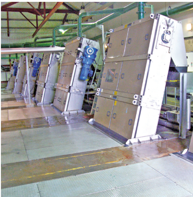
Universally applicable HUBER RakeMax® screen for big channel widths and big discharge heights.
