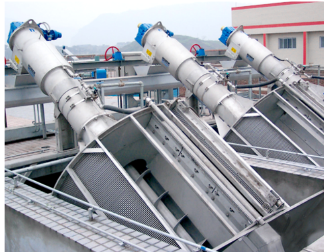
Several parallel HUBER Fine Screen ROTAMAT® Ro1 units installed in the channel.
