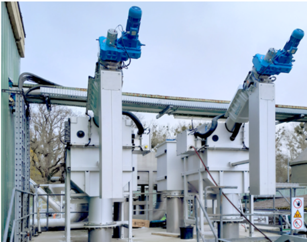
Outdoor installation of HUBER Fine Screens ROTAMAT® Ro1 with heating for frost protection.
