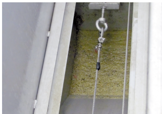
Paddle scraper for grease removal from the grease trap. According to the principle of a longitudinal grit removal scraper the grease paddle pushes the floating fat and grease into the pump sump.
