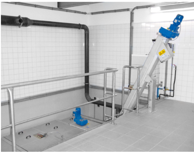
Integrated grit washing at the end of the HUBER Complete Plant ROTAMAT® Ro5.
