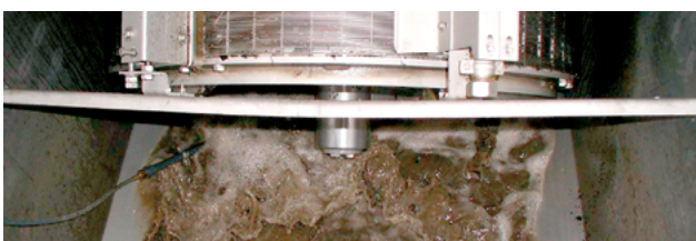
Well-proven wastewater fine screen: HUBER Rotary Drum Fine Screen ROTAMAT® Ro2.
