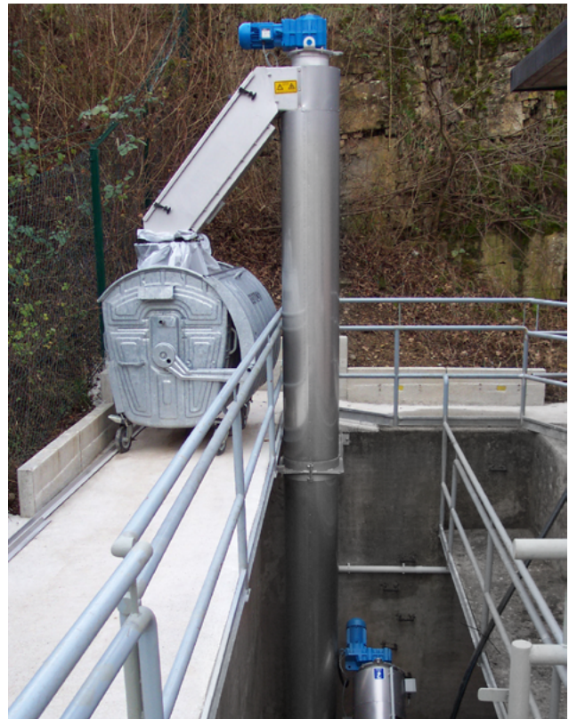
Vertical discharge of screenings from a micro strainer out of a deep manhole.
