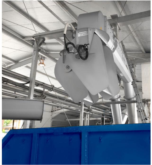
Open distribution chute for screenings in tip mode.
