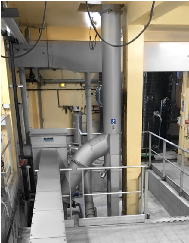
Underground screenings system, vertical wash press discharge with downstream Ro8 V.
