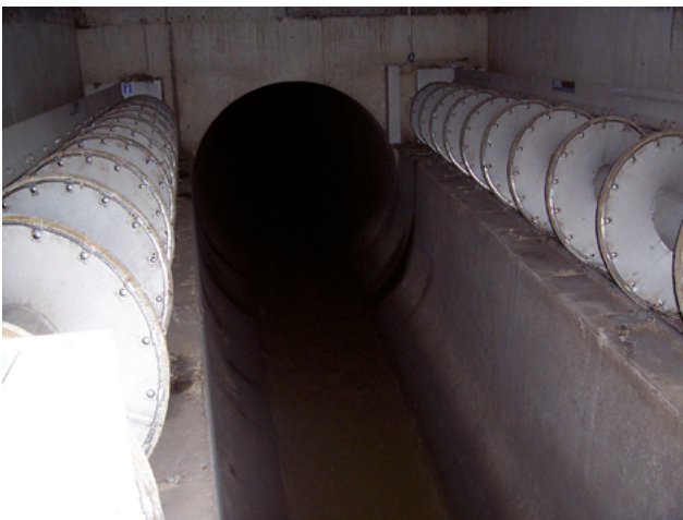
ROTAMAT® RoK1 screens installed at an angle of 60° on both sides of an overflow.
