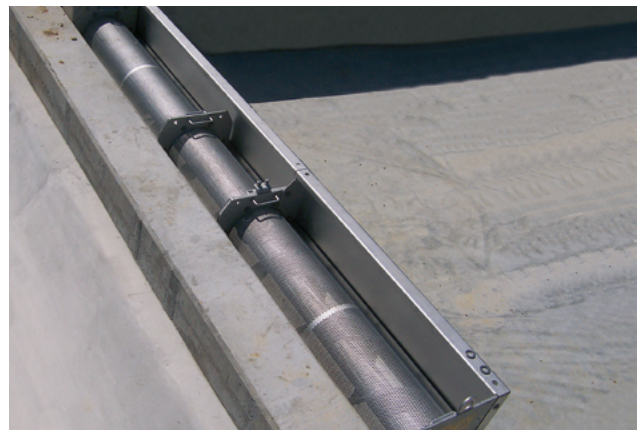
HUBER Storm Screen ROTAMAT® RoK2 after completed installation.
