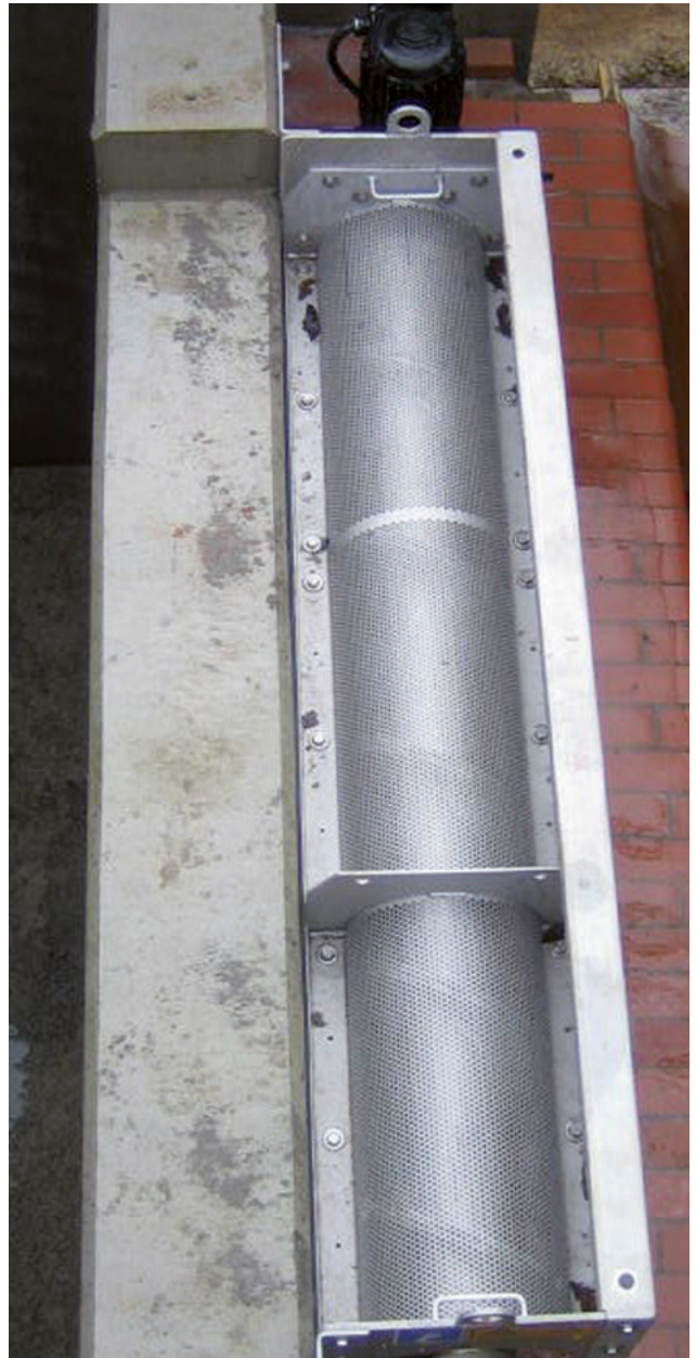
HUBER Storm Screen ROTAMAT® RoK2 installed at a stormwater discharge.
