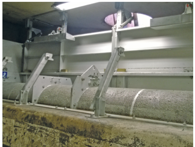
HUBER Storm Screen ROTAMAT® RoK 2 – Optional version with emergency overflow.
