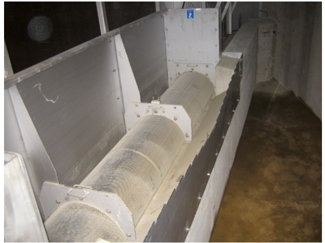
HUBER Storm Screen ROTAMAT® RoK2 with an integrated gauging weir for overflow measurement.
