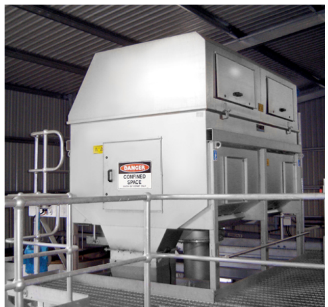
Installation of a HUBER Drum Screen RoMesh® for industrial wastewater treatment.
