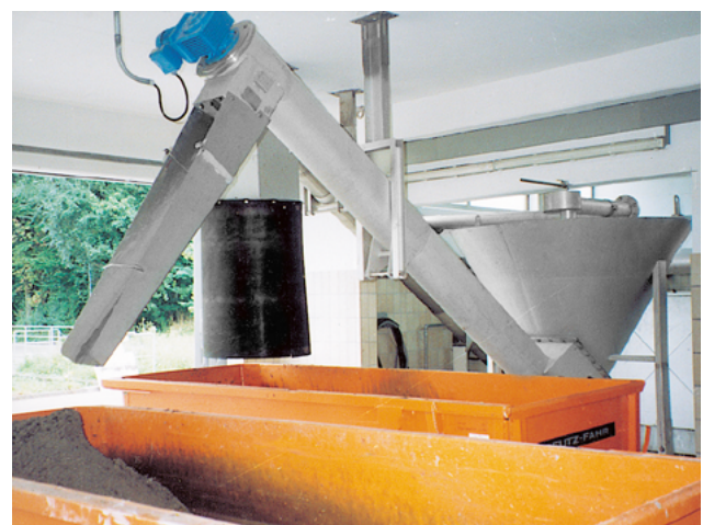
A classifying screw transports the grit from the separation room into a skip.
