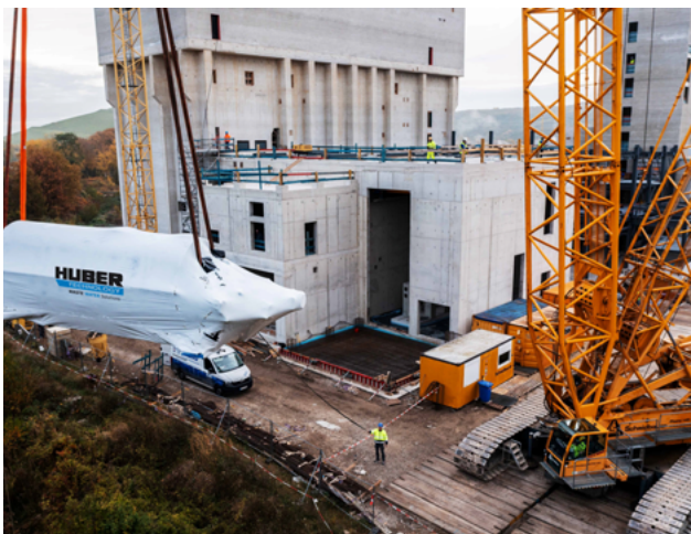
A disc dryer is lifted into place with the help of a heavy-duty crane.
