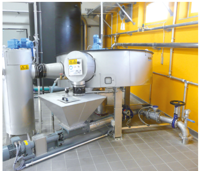
HUBER Disc Thickener S-DISC designed to thicken 35 m 3 /h.
