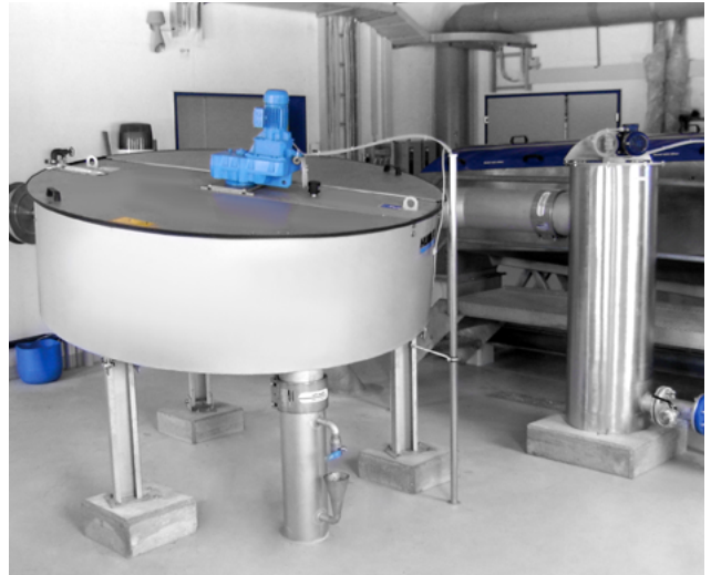
HUBER Disc Thickener S-DISC size 2 with preceding flocculation reactor.
