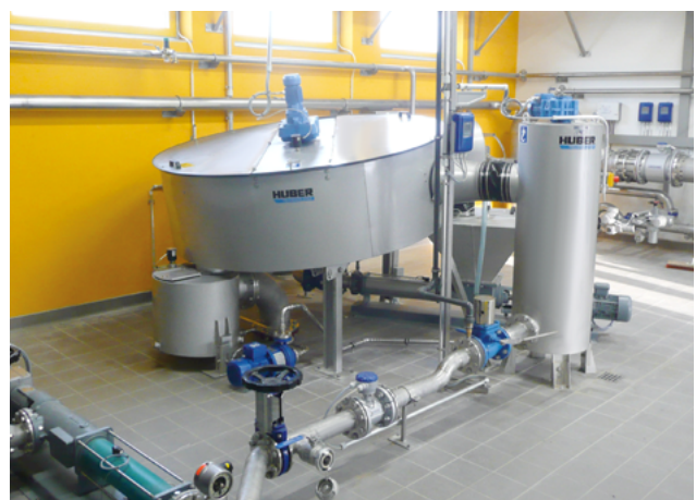
Filtrate storage tank and spray water pump for water recycling.
