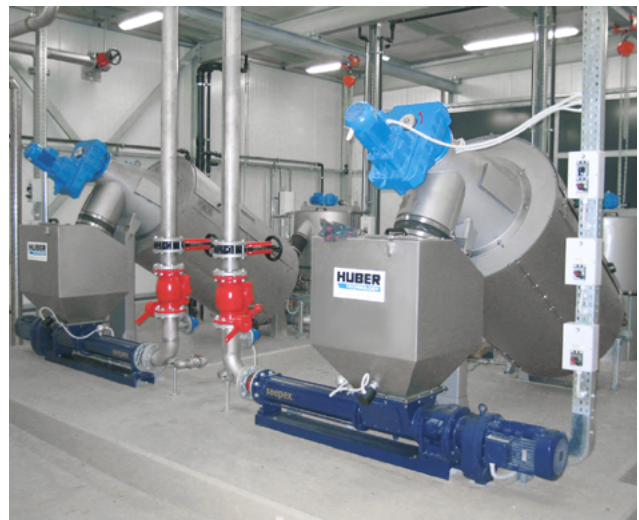
Two HUBER Rotary Screw Thickener S-DRUM units for 80 m³/h.
