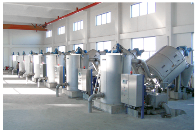
Eight screw thickeners handling 600 m³/h.
