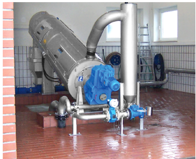
HUBER Screw Press S-PRESS for 8 m³/h.
