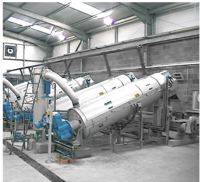
Parallel installation of six HUBER Screw Press S-PRESS units.
