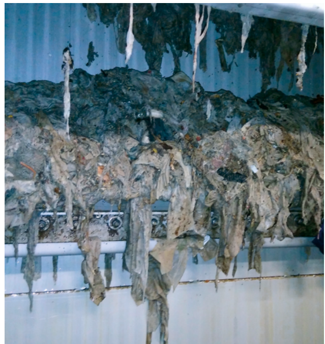
Figure 3: High pollution load on a rake bar.
