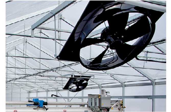
Recirculation air ventilators ensure improved evaporation.
