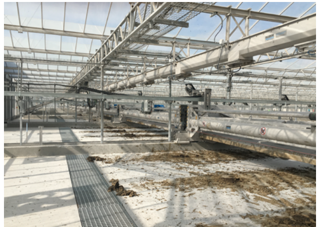
The screw conveyor installed in the floor collects the dry sludge.
