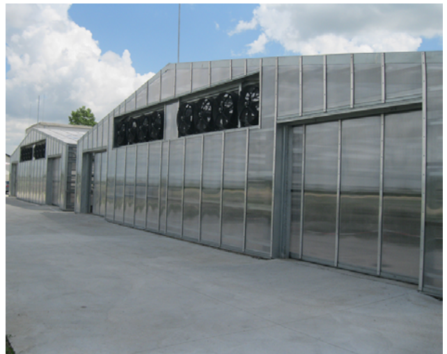
Exhaust fans remove saturated air from the drying halls.
