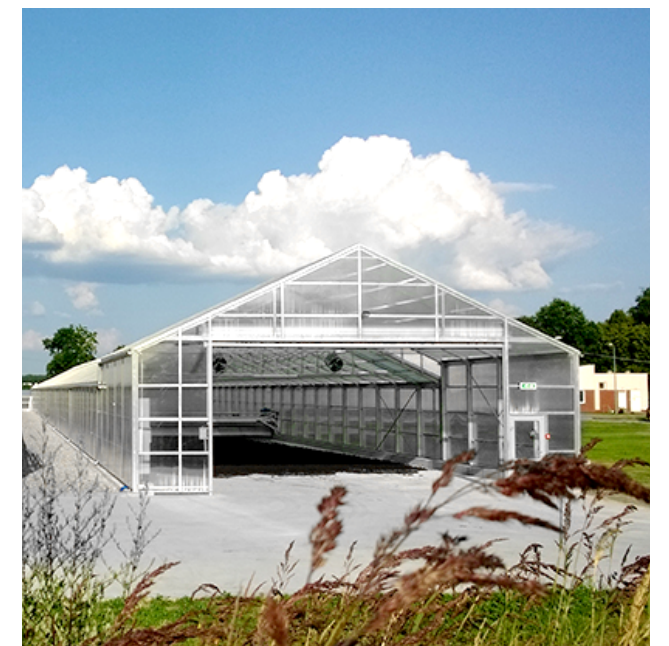
Dewatered sludge is transported in through gates.
