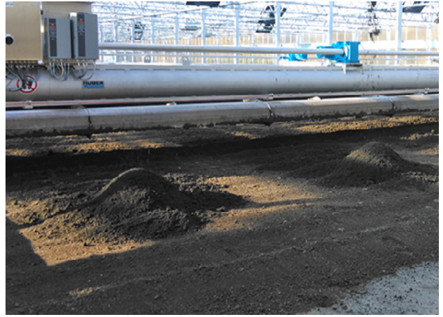
Automated sludge feeding with screw conveyors.
