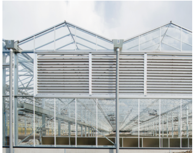
Fresh air enters the drying hall via weather louvres.
