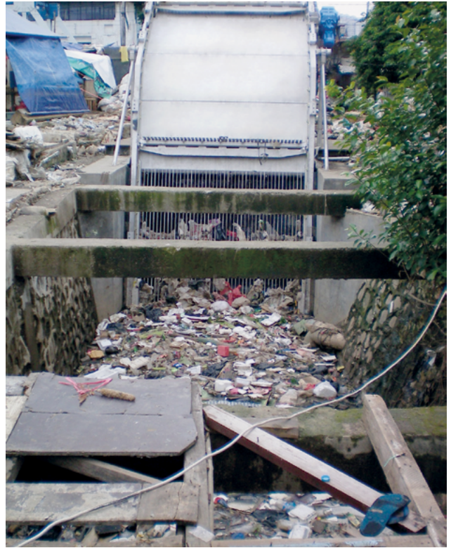
HUBER Coarse Screen TrashMax® in operation.
