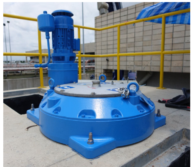
Reliable bull gear drive for the stirrer with airlift.
