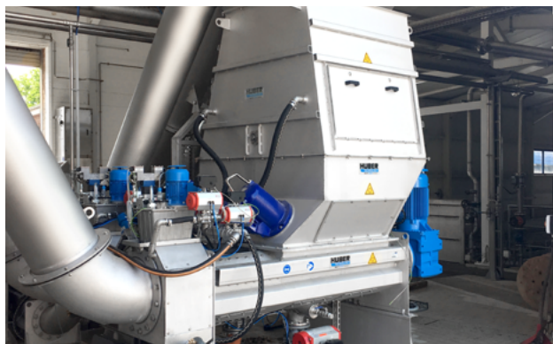
The hydraulic high-pressure unit at the end of the wash press guarantees a maximum DR.
