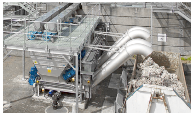
Washed and almost odourless screenings from a HUBER Screenings Wash Press WAP® SL.
